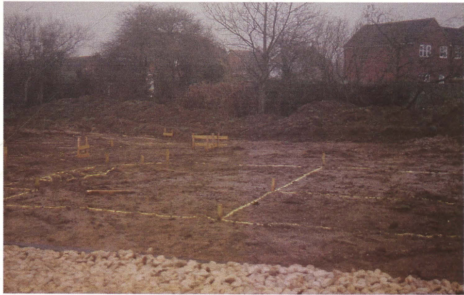
Plate 1 General view plot 5 prior to excavation, looking east
