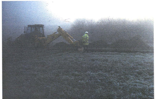
Plate 2: Machining in progress
