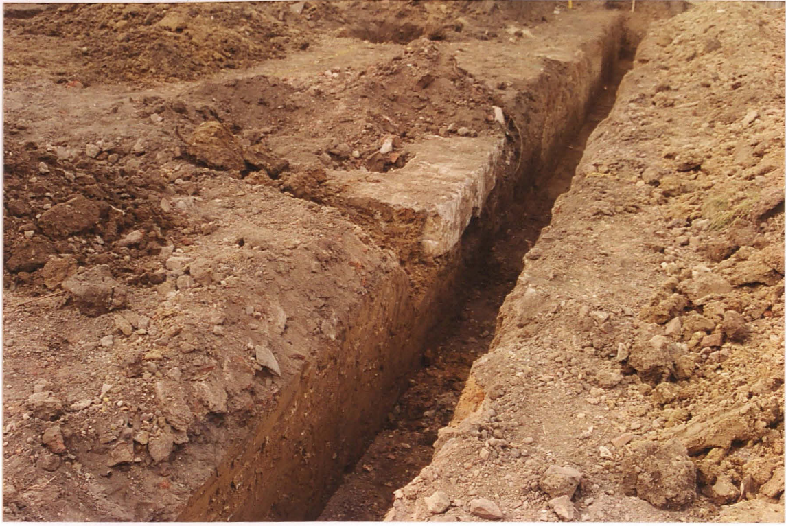
Pl. 7 Dark fills of pits visible in the western face of a north-south foundation trench, below the later concrete slab and at the far end of the trench (looking NW).
