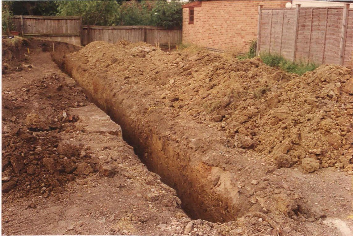
Pl. 8 Eastern face of a foundation trench, with soil colour variations marking the positions of pits and later disturbances (looking NE).
