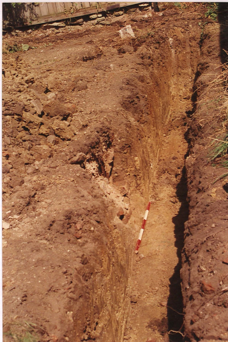
Pl. 11 Position of the brick-lined feature 5 in the eastern foundation trench (looking north; scale 1m). The stone wall foundation marks the boundary with Octavia Cottage, behind the new development.
