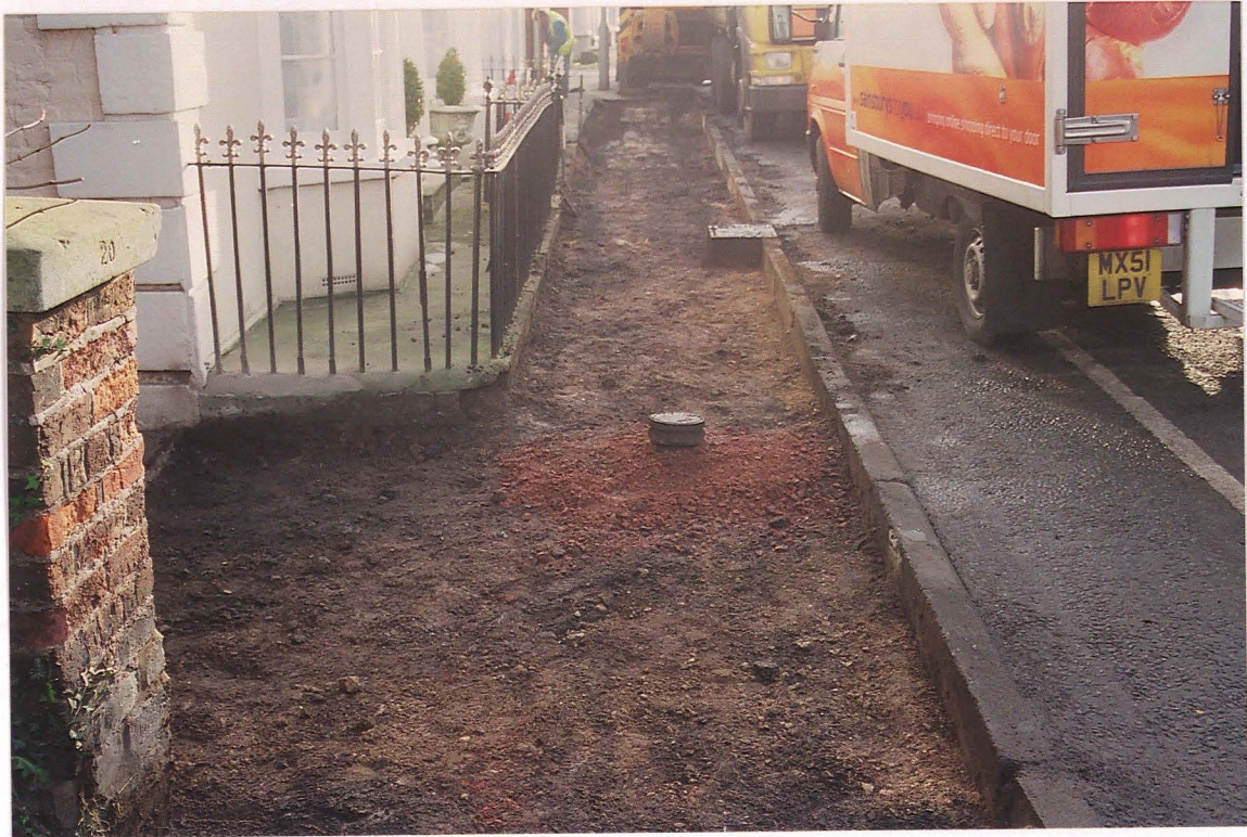
Pl. 2 The tarmac path surface was removed alongside Market Street (looking east).
