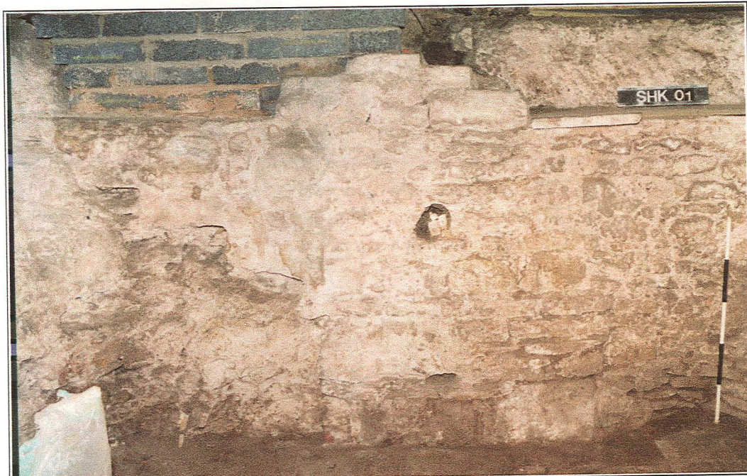
Plate IV – Block of limestone in east wall of cellar (looking east, 1m scale).
