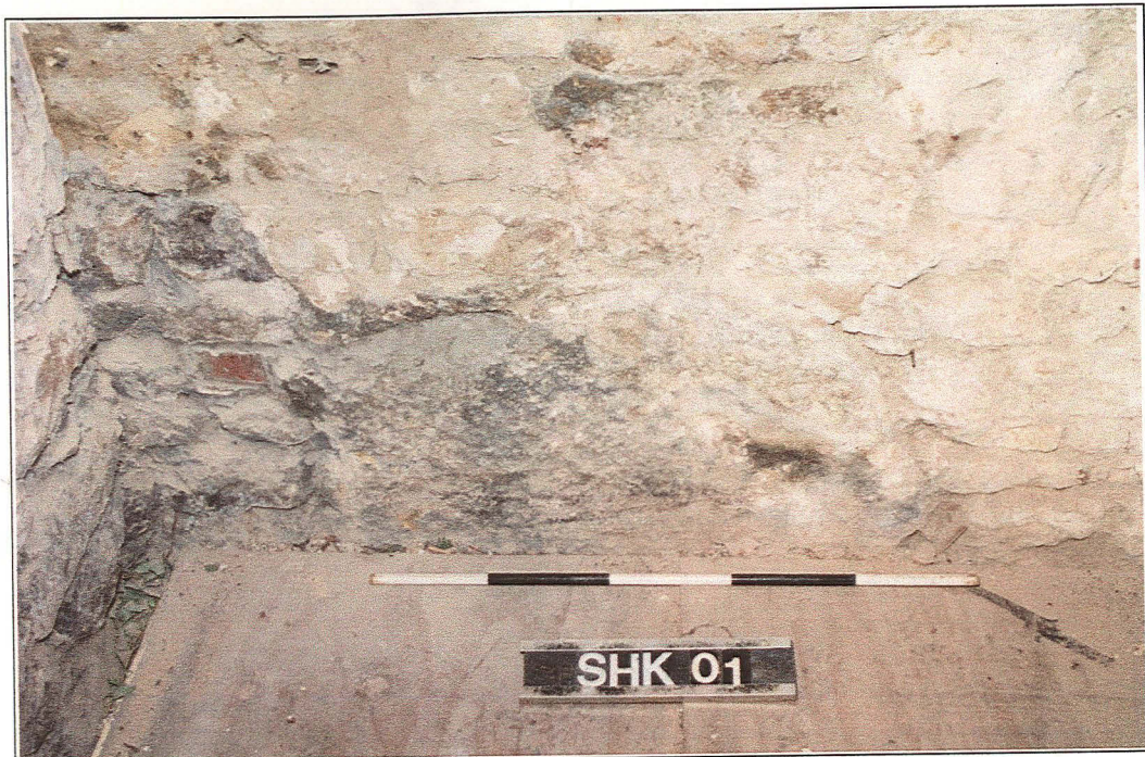
Plate III – Block of limestone in south wall (looking south, 1m scale).
