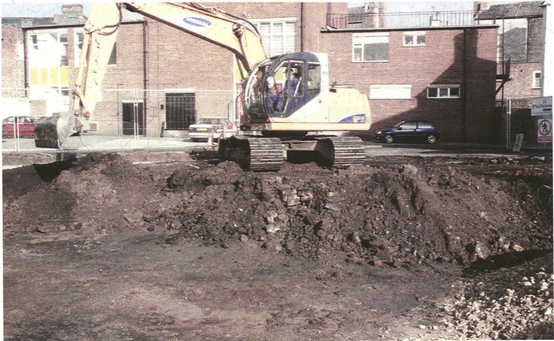
Plate 1 General view excavation area looking east
