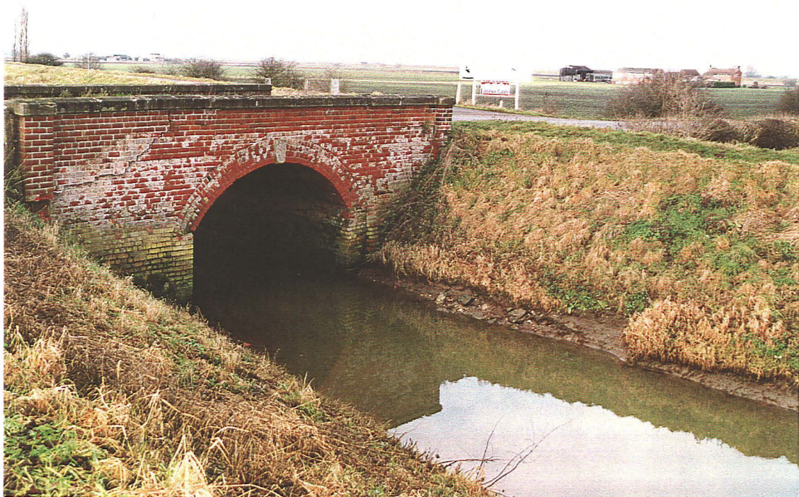
Plate 4: Section (39) – brick bridge carrying Causeway Road over the Billingham Skirth, looking north-west. Note the concentration of limestone rubble visible at the waterline c. 2m to the east of the bridge.
