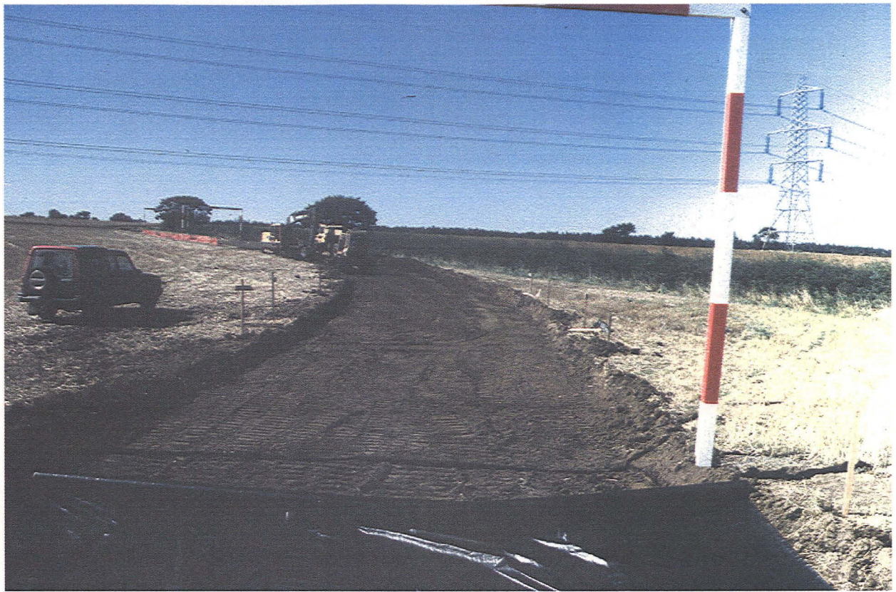
Plate 1: View of stripped area along access road
