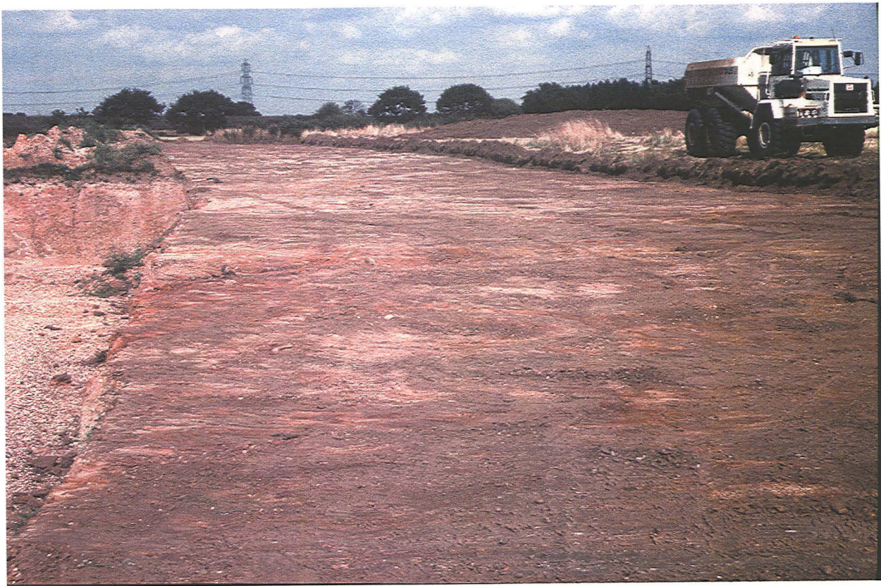
Plate 3: Initial stripped access route within mineral extraction area, looking east
