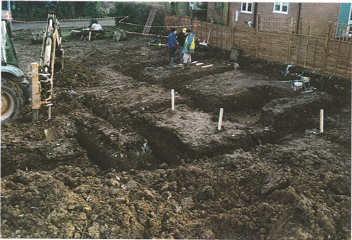
Plate 5: General view of footings trenches, looking S.
