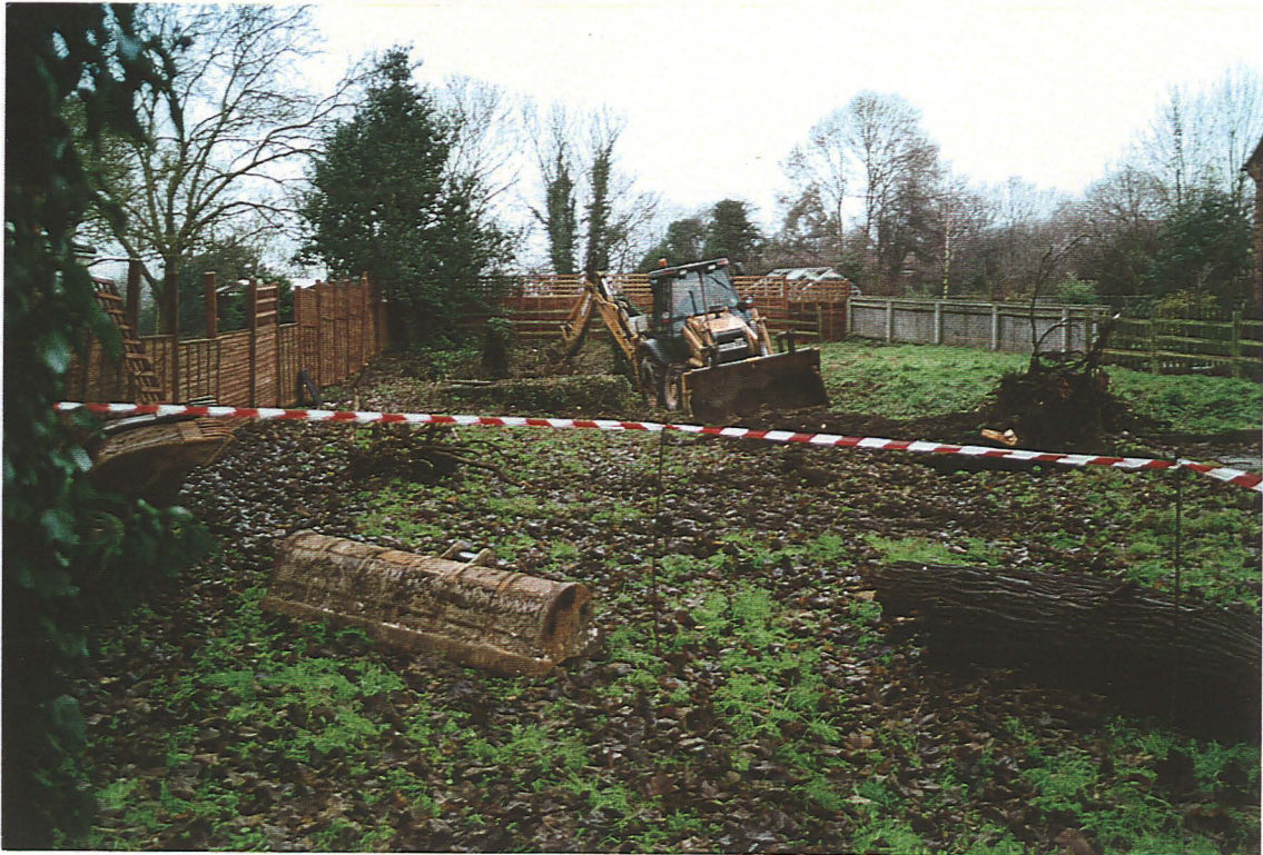
Plate 1: General view of the site before ground clearance, looking NW
