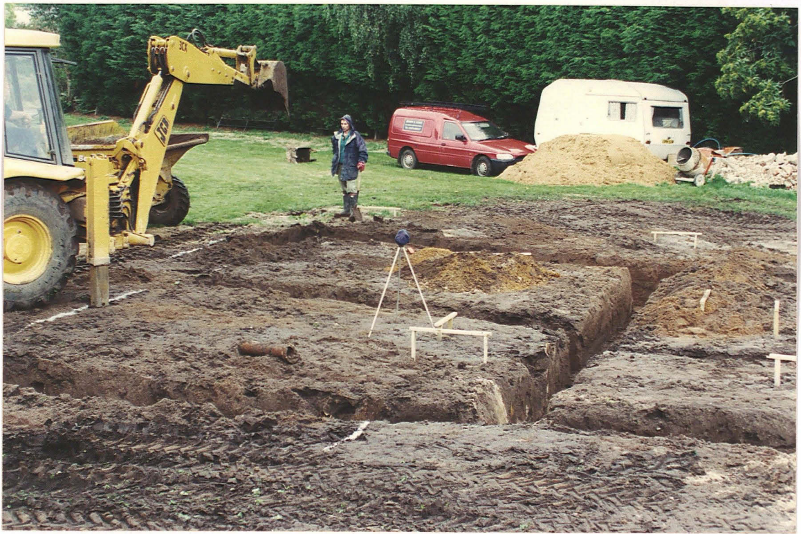
Pl. 7 House plot foundation trenches, looking north-west.
