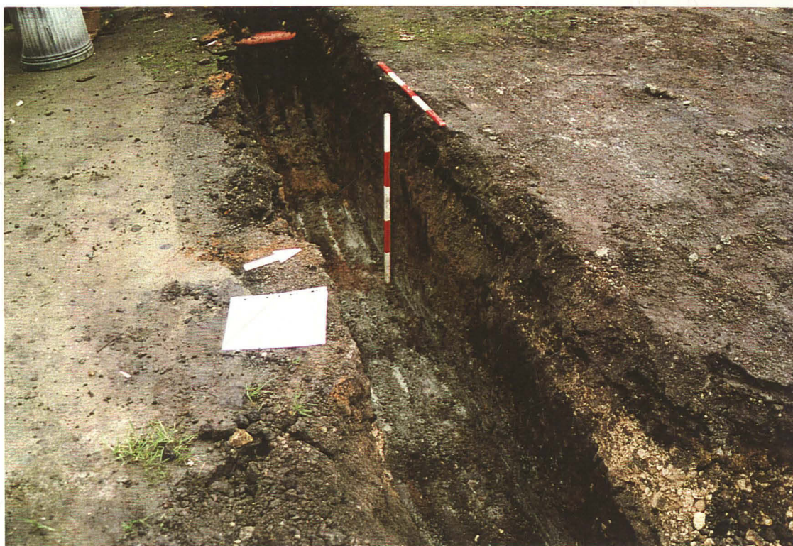
Plate 3. Foundation trench for the south wall of the extension, looking NW.
