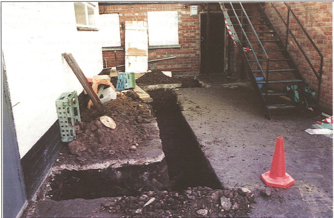
Plate I: General view of the foundation trench (looking west).
