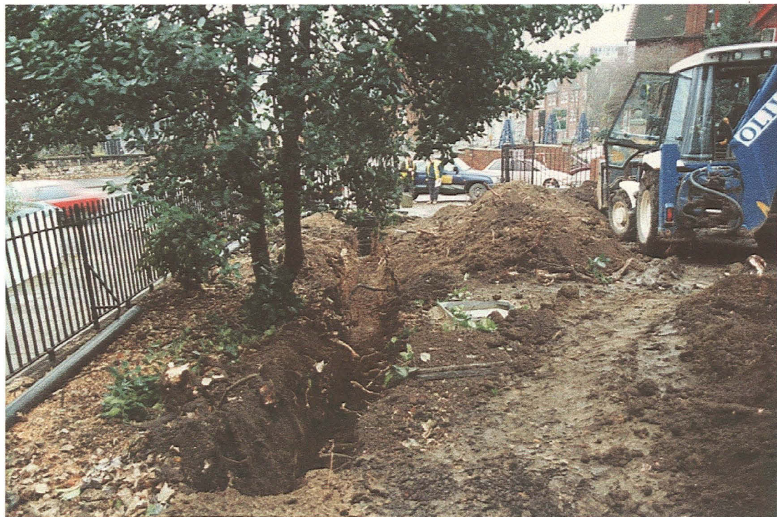
Plate 2: General view of cable trench along eastern site boundary - looking south
