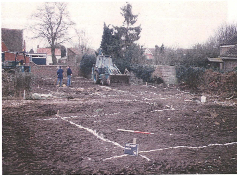
Plate 1 - General view of the development area, looking northeast
