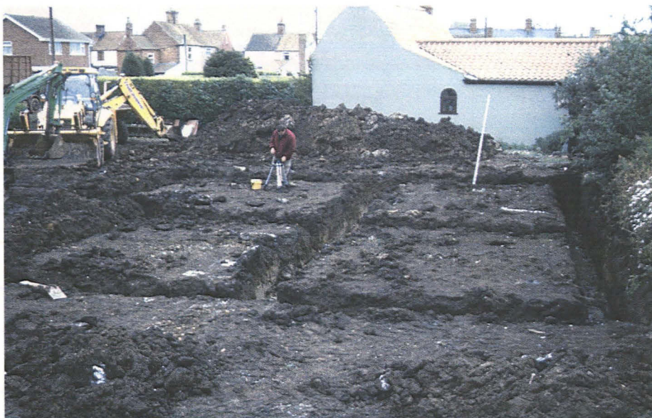
Plate 1 General view of the development, looking west.
