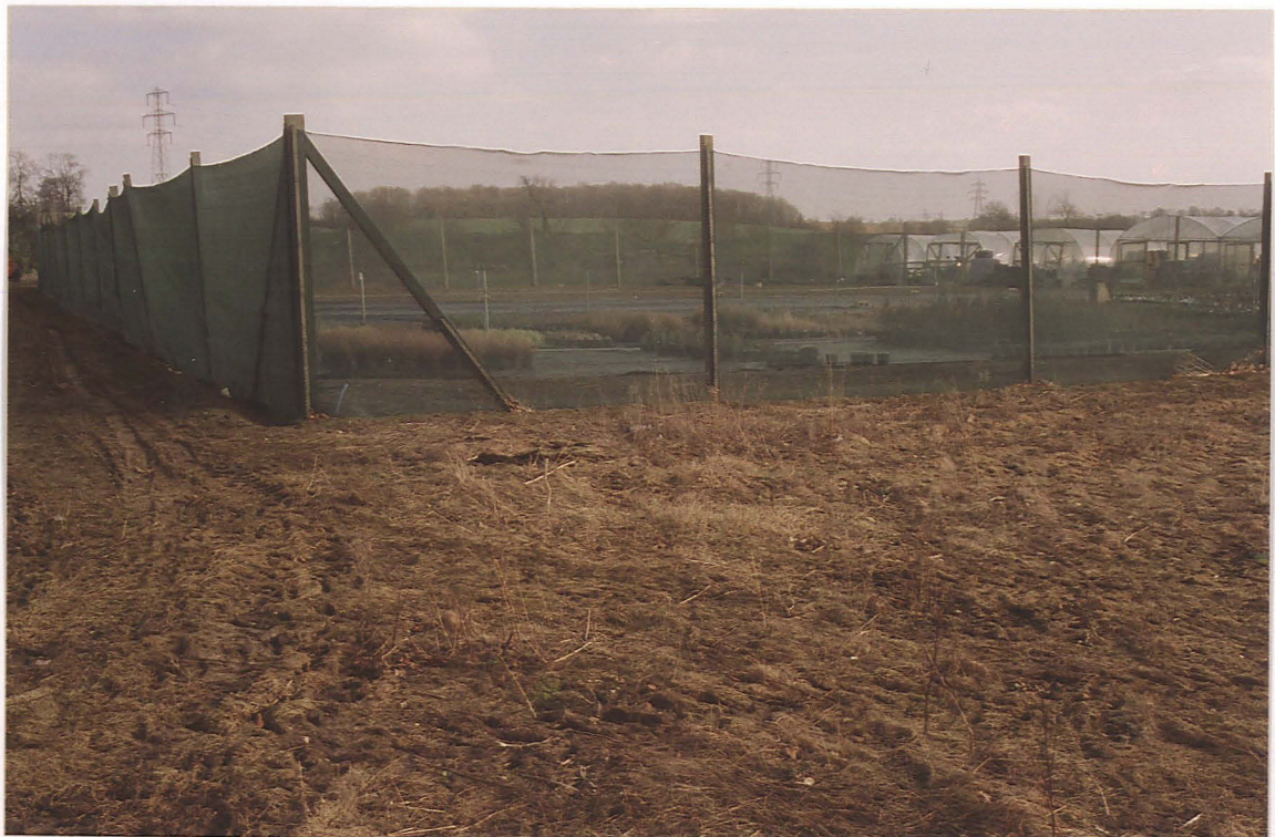
Pl. 8 Windbreak structure within the application site (looking NW).
