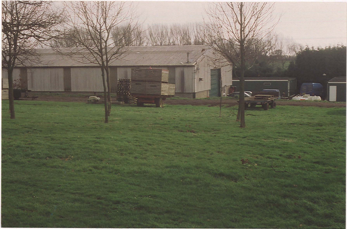
Pl. 3 The existing sports hall and adjacent temporary buildings, cut into the natural slope (looking NW from parkland).
