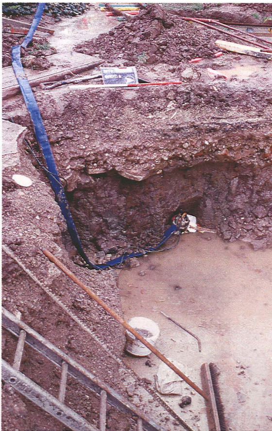
Plate 3 General view groundworks (Section 6) Stanchion pit F12B
