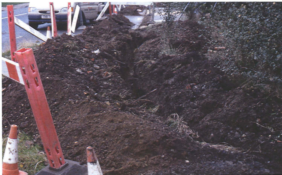
Plate 3 General view work in progress area 2
