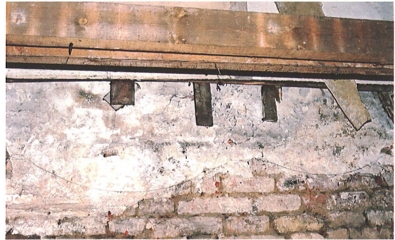
Plate 19: Room Bi; bases of Phase III stud partition
