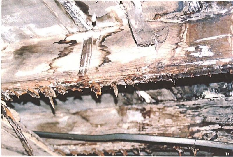
Plate 25: Ceiling joists of Room C showing ovolo scratch moulding
