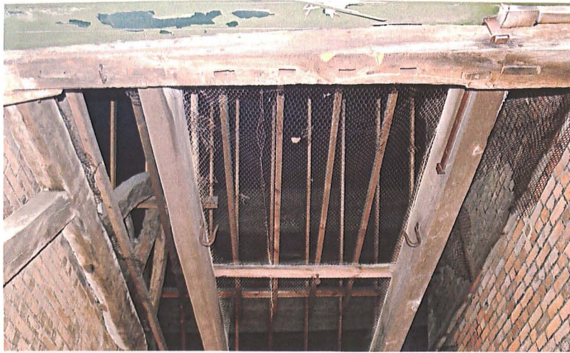
Plate 17: South wall plate over Bay 3 showing mortices for wooden mullioned window
