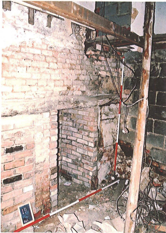
Plate 18: Room B; Phase II brick chimney showing oak lintel
