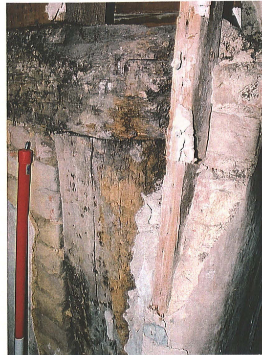
Plate 16: Principal post of Frame B exposed at top of current stair
