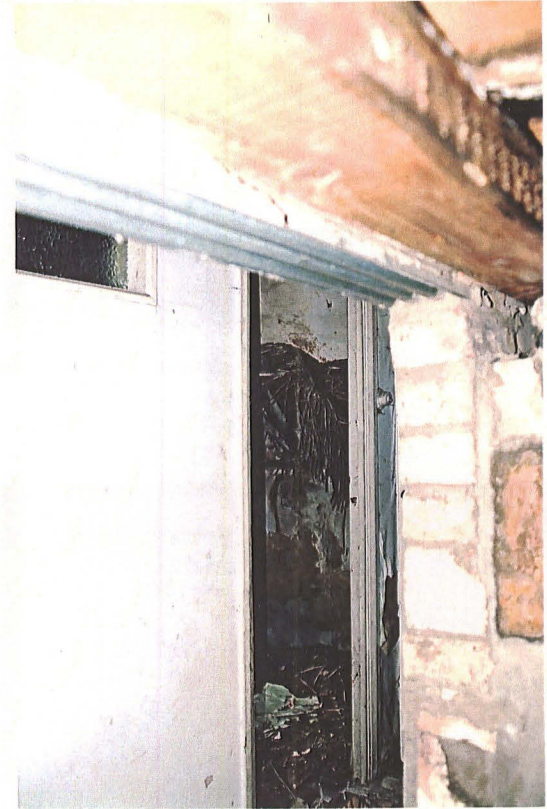
Plate 27: Thatch course or fleeking seen through doorway through to Room Ci
