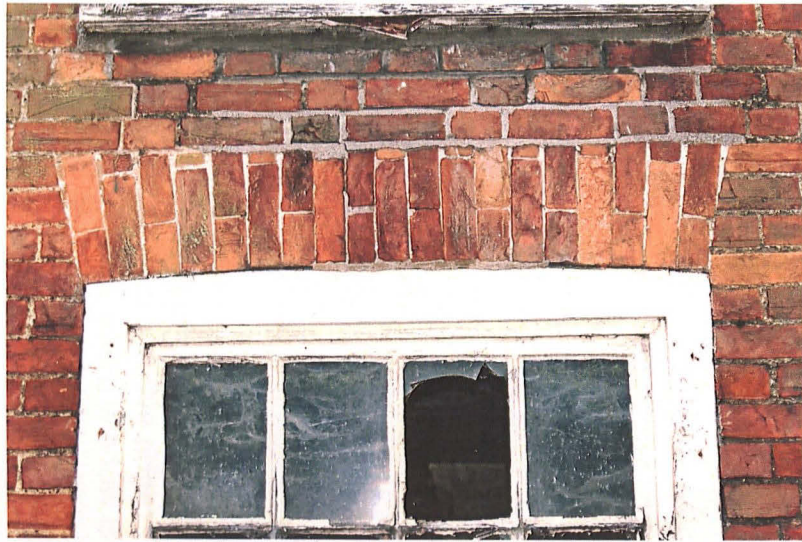
Plate 28: Detail of flat-camber window arch of No 11 East Street
