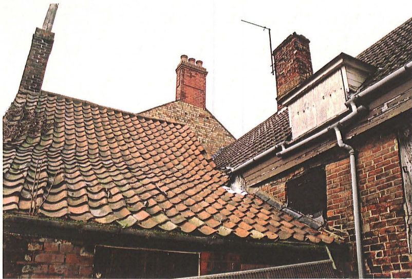
Plate 26: Roof detail of Phase IV/A/B
