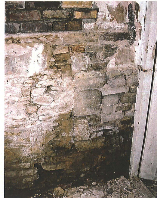
Plate 3: Detail of change in build of stone pinning
