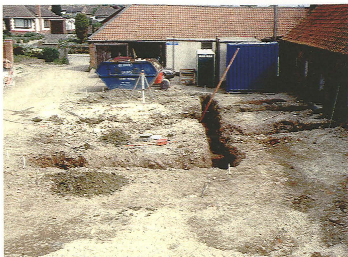
Plate 4 - View across Plot B1 showing the former barn, looking north
