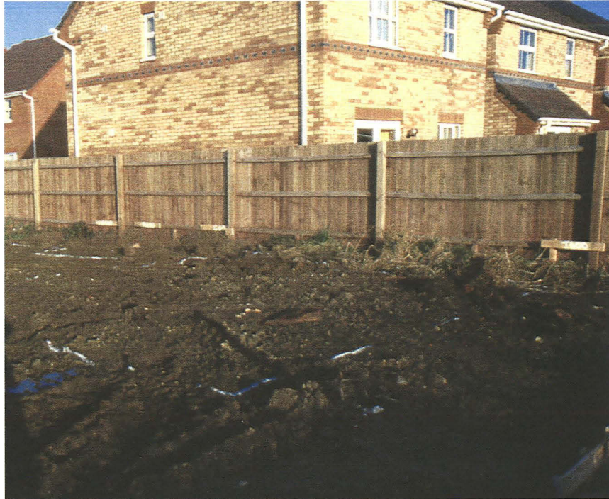
Plate 1 General view of site at commencement of groundworks, looking north
