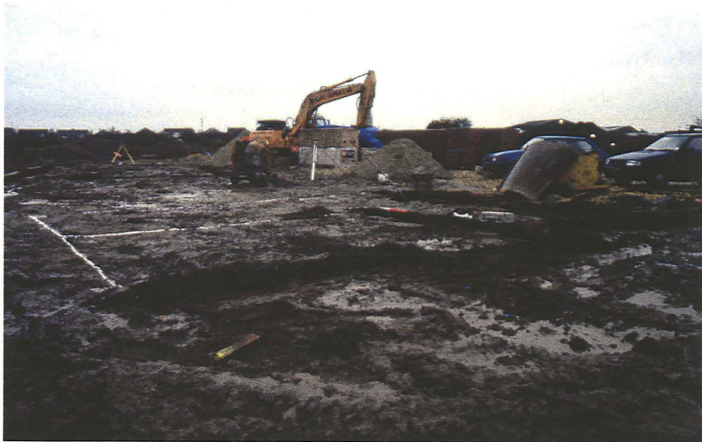
Plate 2 General view plot 24, looking north
