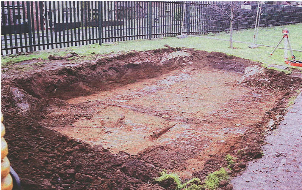
PL 1: General view of the site, looking north-east
