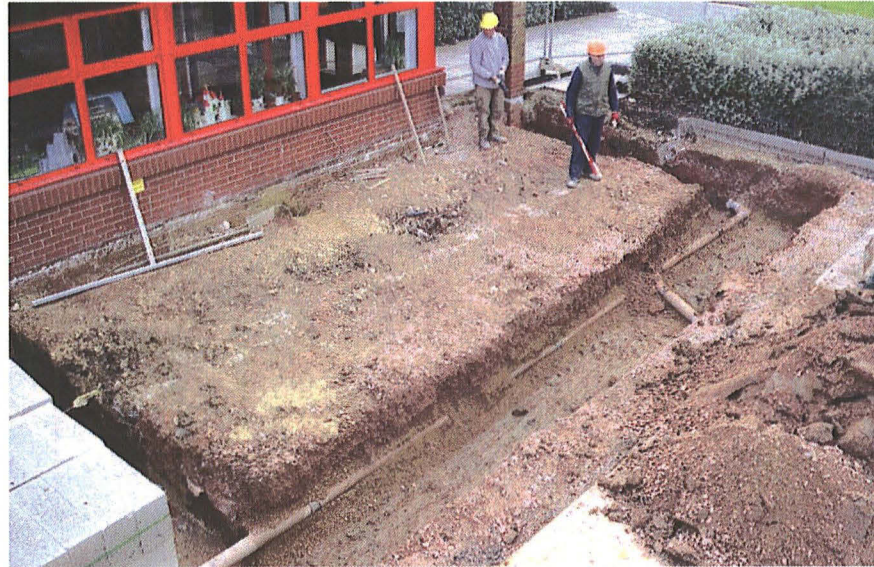
Pl.1: General view of the site, looking south-west
