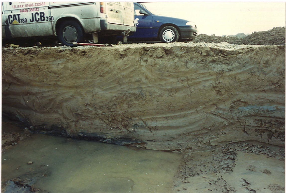
Pl. 5 Ditch 179 cut the blue/grey silt band 183 (right), interpreted as a medieval or early post-medieval topsoil. Looking south.
