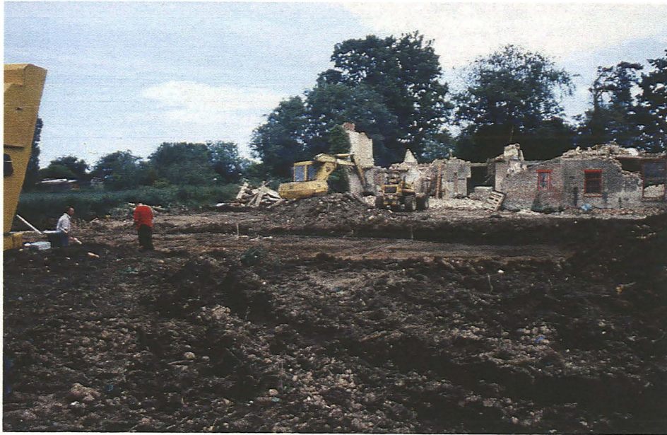
Plate 1 General view of site showing remains of Old Rectory
