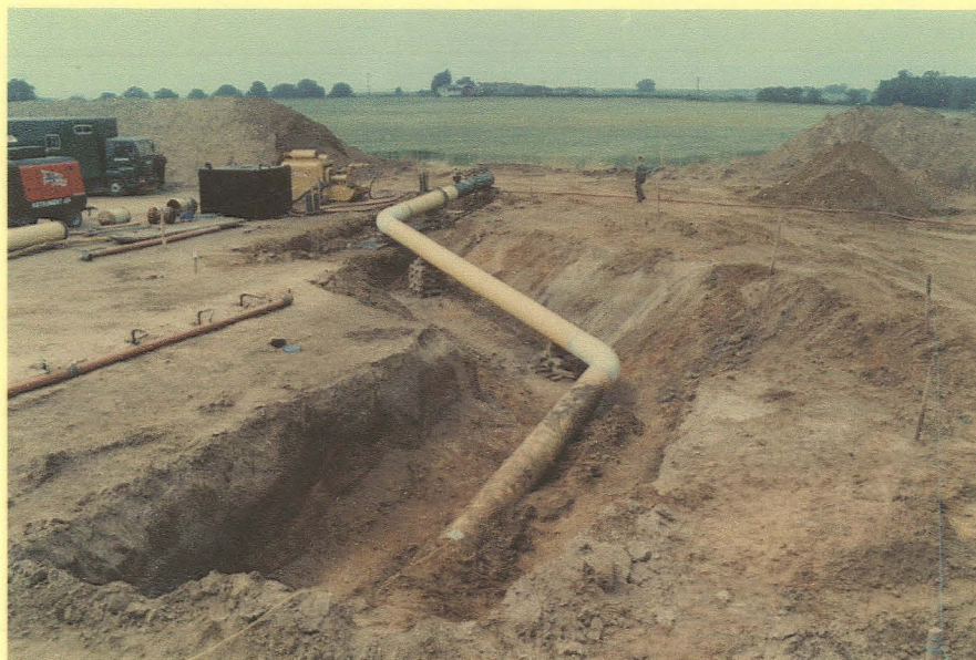
(Area 4 pipe cutting, photograph by R.Holt)
