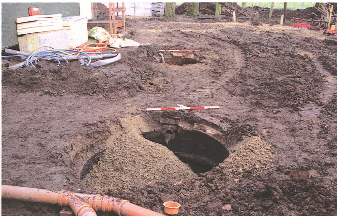
Plate 2: General view, looking north-east across the footprint of the new classroom, Victorian cesspit [005] is in the foreground and soakaway [006] can be seen behind.
