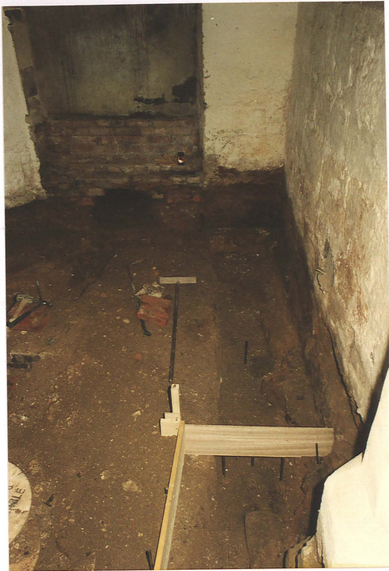
Pl. 5 Service trench dug along tower north wall, looking west.
