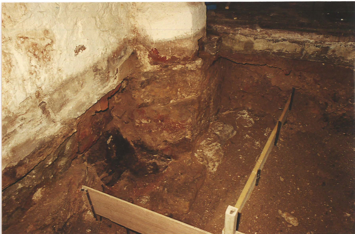
Pl. 6 Polygonal base of tower arch (north side) resting on foundations for tower north wall.
