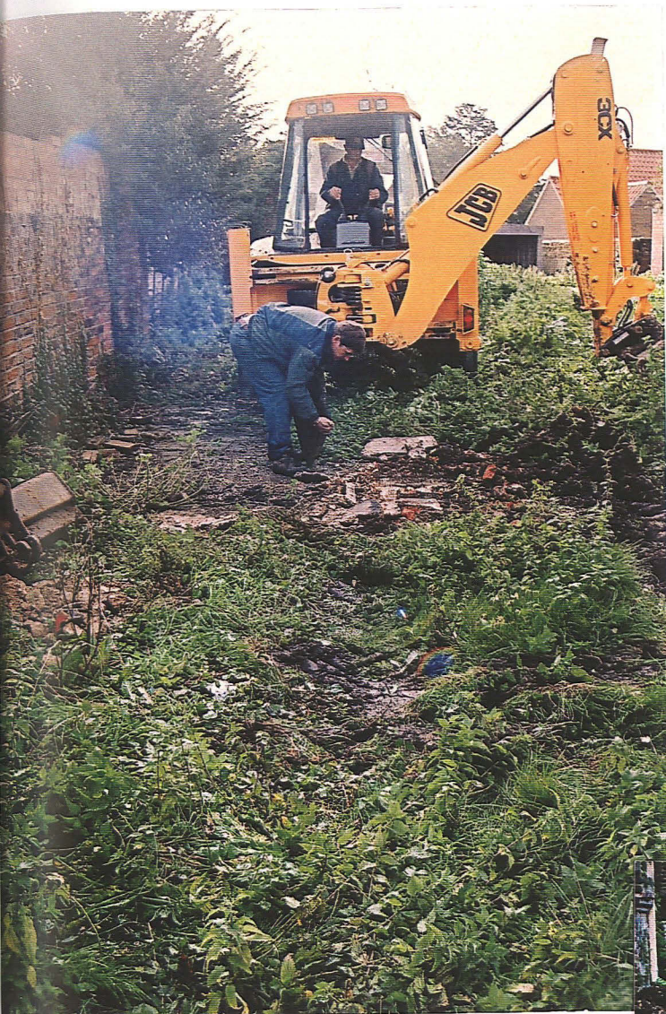
Plate 1. The site prior to trenching
