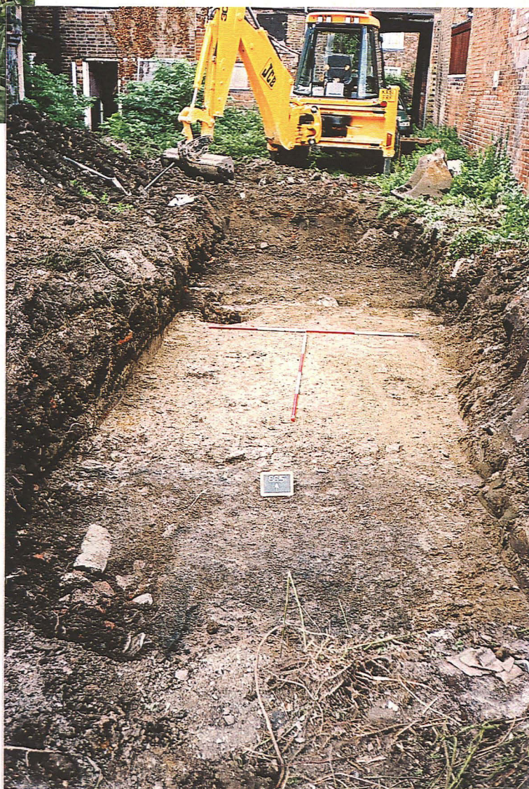
Plate 2. The trench after machining and cleaning showing context (015) in the foreground
