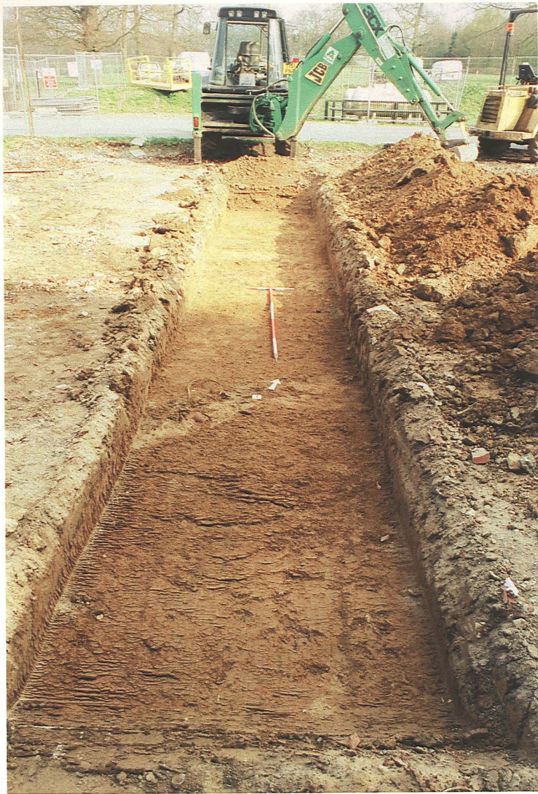
Pl. 3 Trench 1 (right) scales 0.50m and 2m
