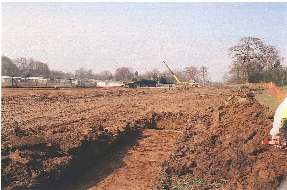
Pl. 2 General view looking east from Trench 4
