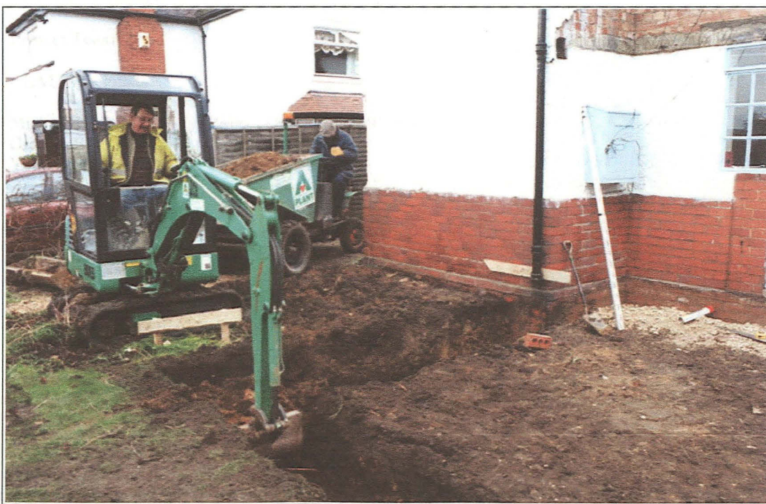
Plate I: General view showing the machine excavation of the foundation trench for the rear extension (looking north).
