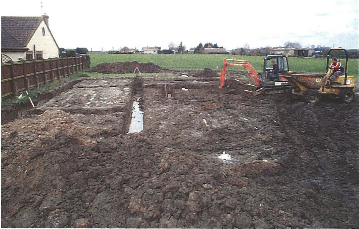
Plate 1: General view of site with work in progress, looking west
