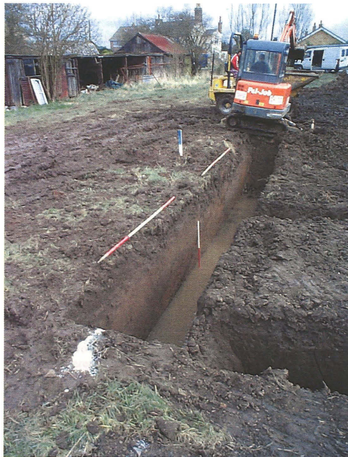
Plate 2: View of Section 3, looking northeast
