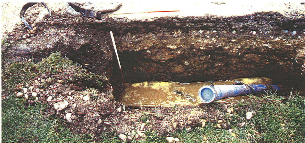
Plate 2 Section 1 in Pit 1 (Area 1) looking south
