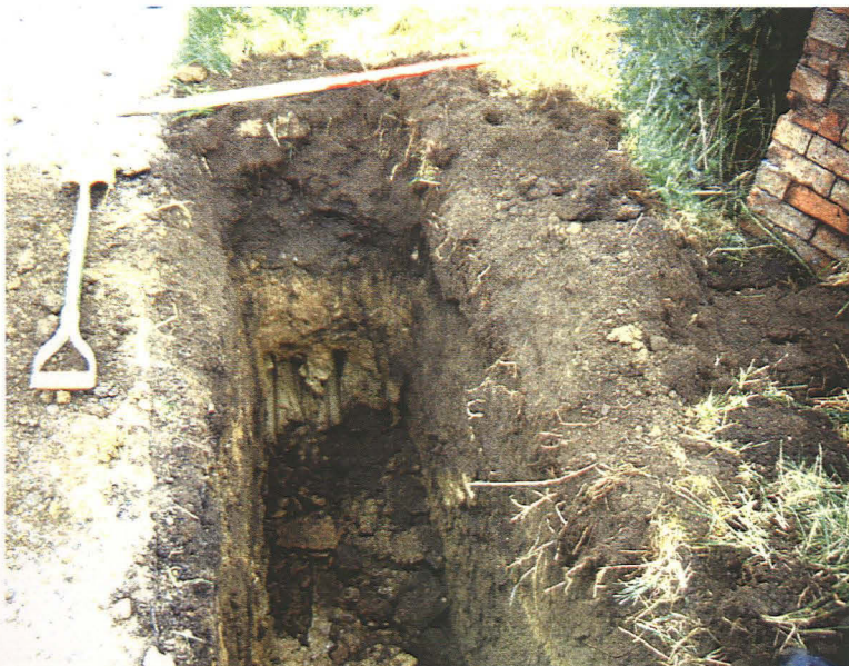
Plate 3 Section 4 in Pit 7 (Area 2) looking north
