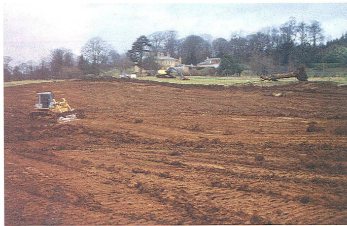
Plate 2: Groundworks with Dalby Hall in background (looking north-west)
