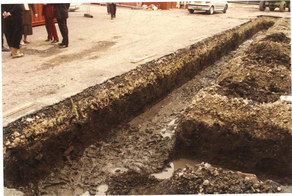
Pl. 4 Brick cover of tile drain visible to east of Trench 2 in the eastern face of Trench 8 (looking SE).
