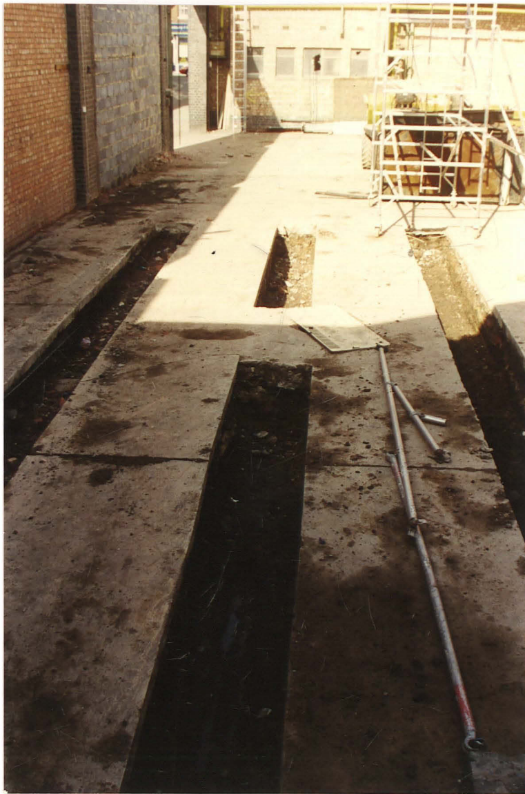
Pl. 13 Position of the three narrow slot trenches in Cinema 1 (looking north).
