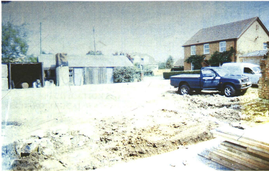
Plate 1 General view of site prior to groundworks, looking northeast.
