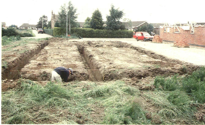
Plate 1 - General view across the development area, looking southwest
