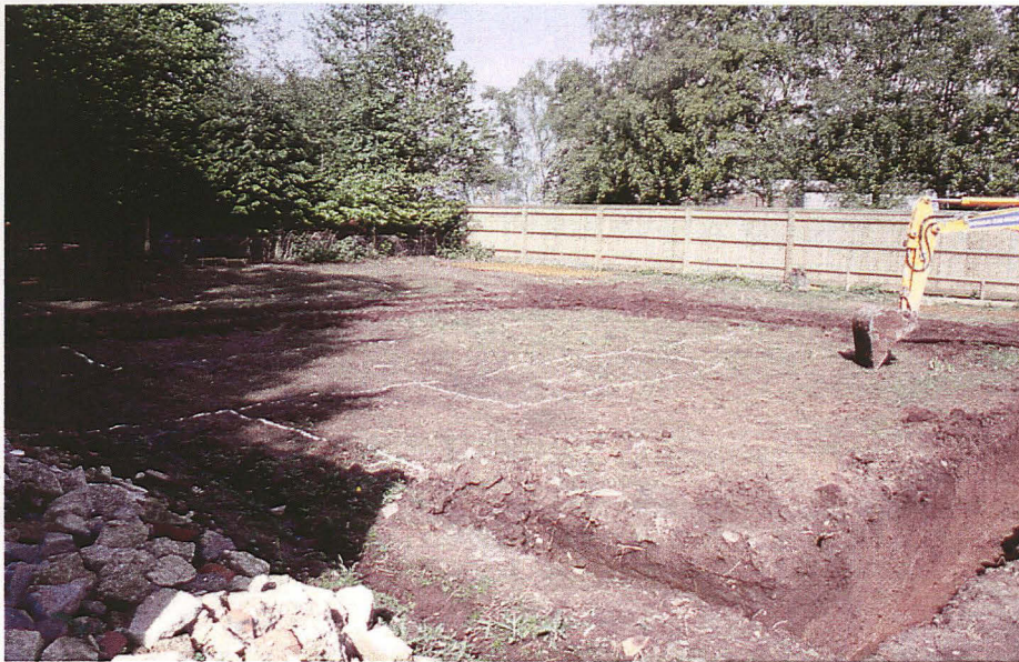
Plate 1 General view of site during groundworks
