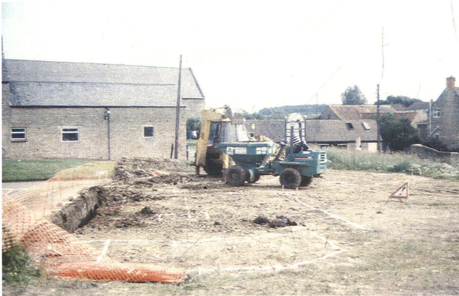
Plate 1 General view of site, looking north.
