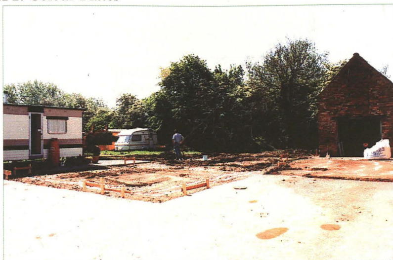
Pl. 1: Site location shot showing foundation trenches under excavation, looking south-east.
