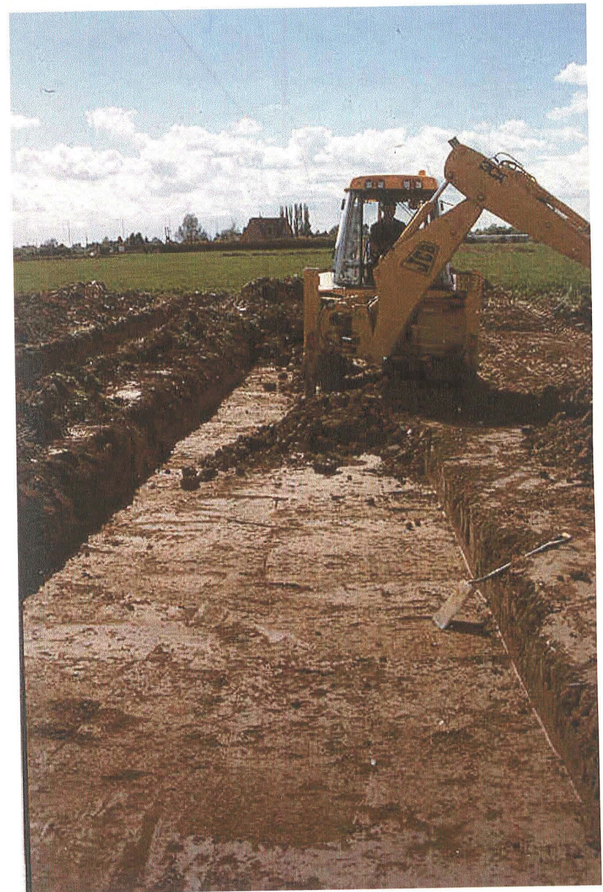
Plate 1: Excavation of the open area
