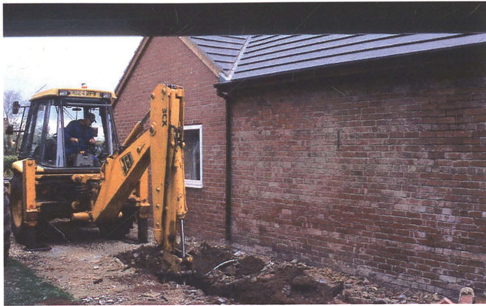
Pl. 1: Excavation of trial trench. Looking north.
