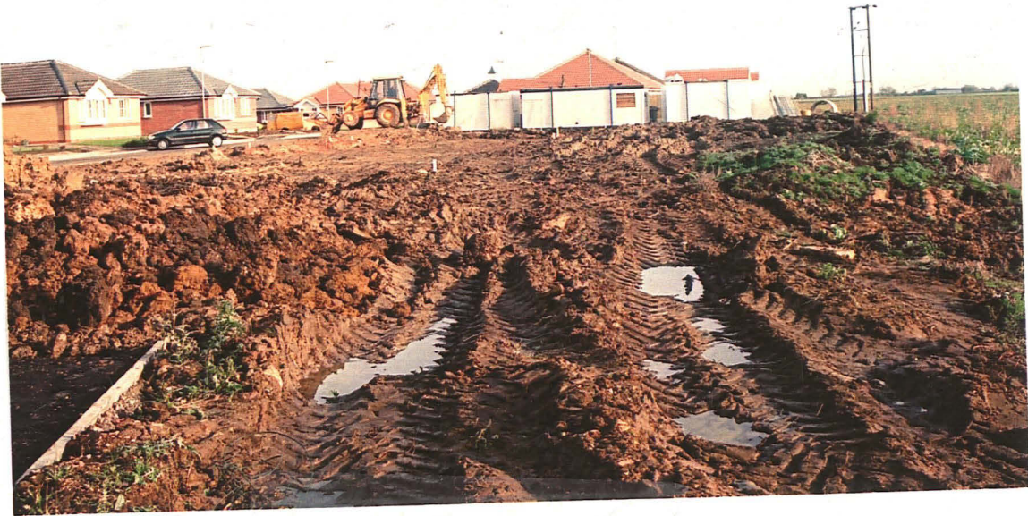
Plate 1. Site prior to groundworks
