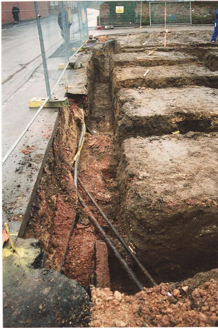
Pl. 18 Service trench running through Plots 12 - 14.
