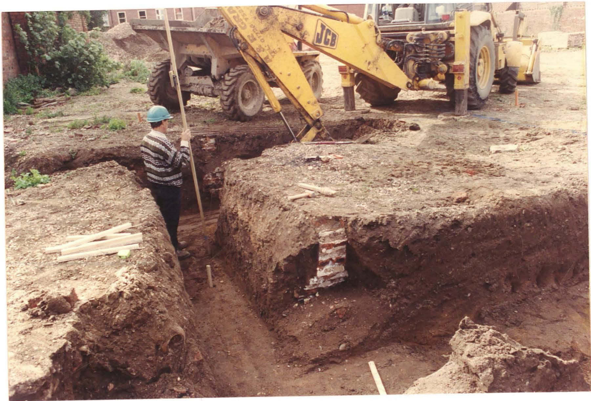
Pl. 11 Footings 502 seen in Plot 7. Looking south.
