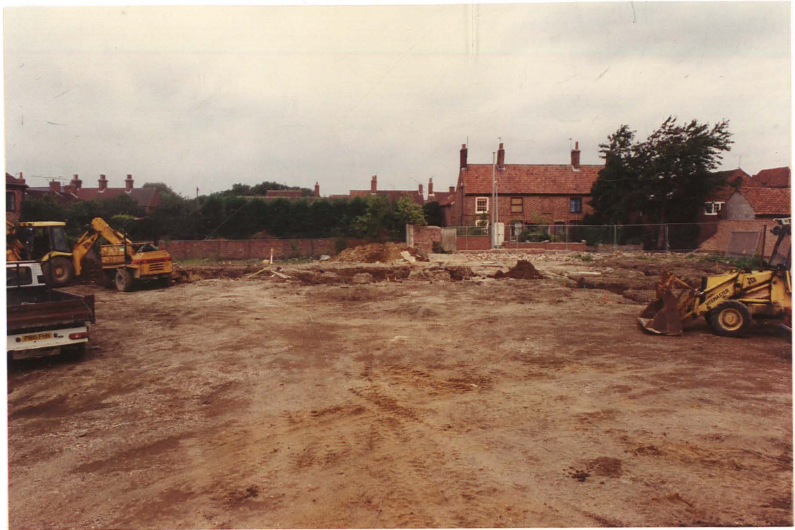
PI. 1 General view of site looking north (Plots 1-4 centre, Plots 5-7 right).
