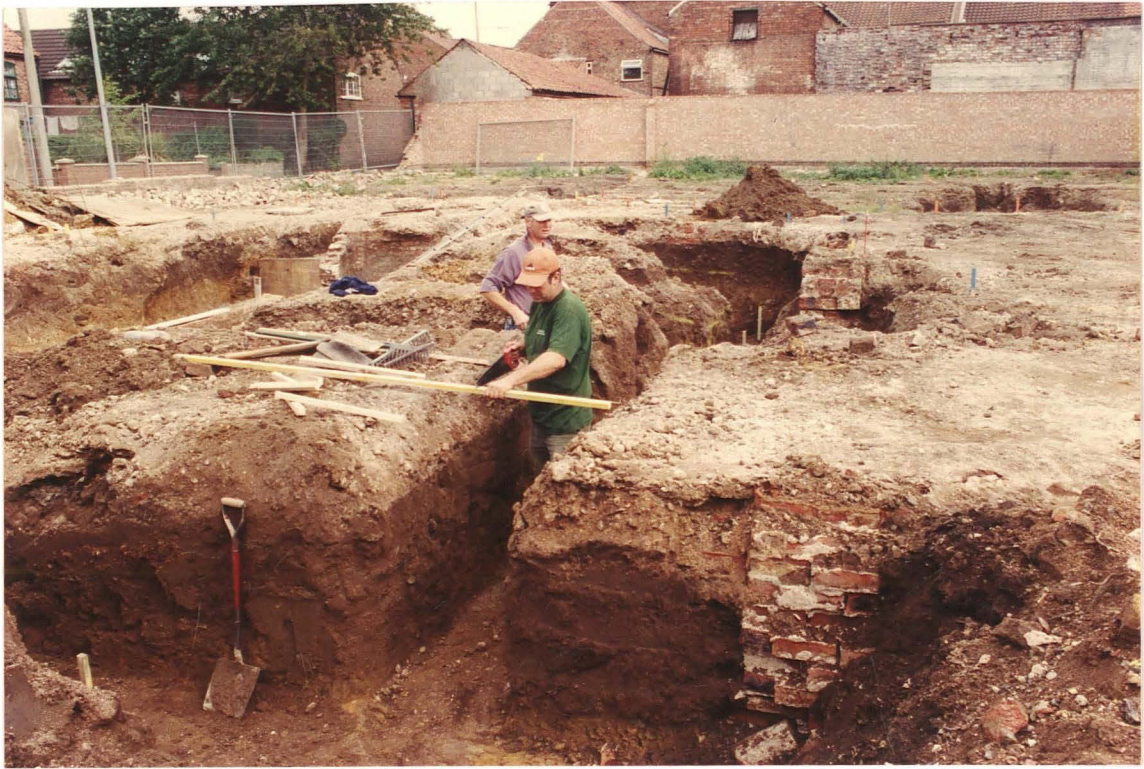
Pl. 7 Plots 3 and 4, south wall foundations of Paddock House.
