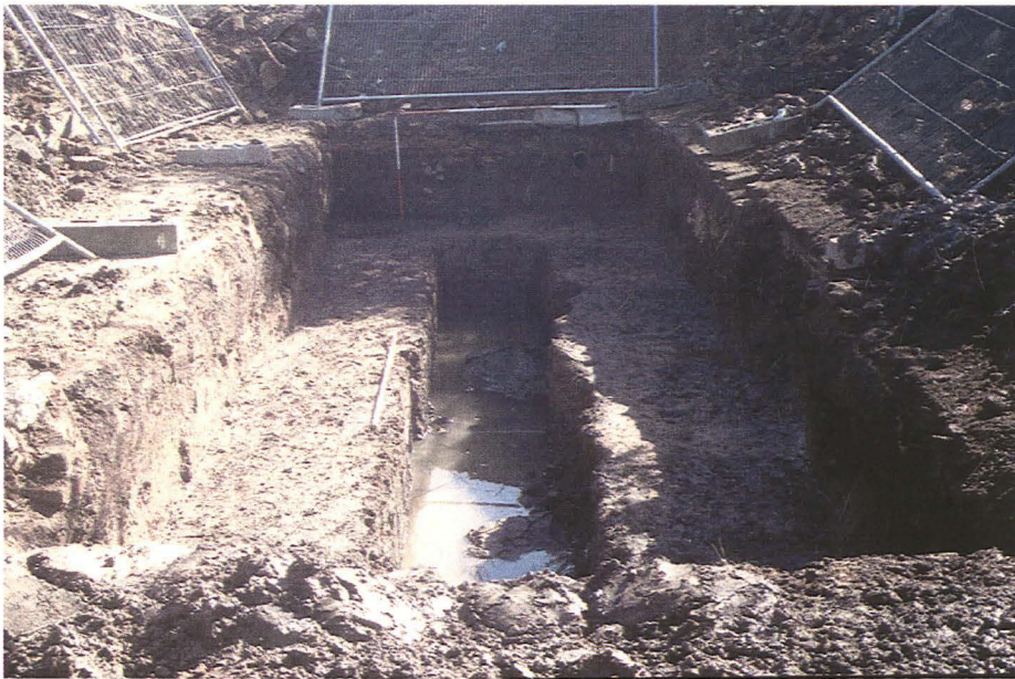
Plate 2: General view of the trench, looking east
