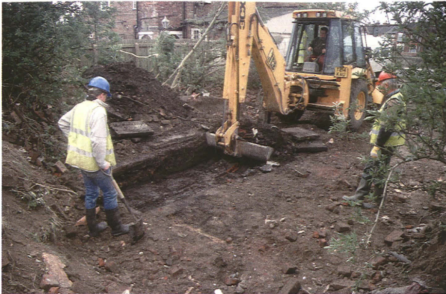
Plate 1: Mechanical excavation of the trench, looking southwest
