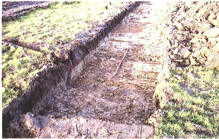
Pl.4: Trench 2, pre-excitation, looking north-east
