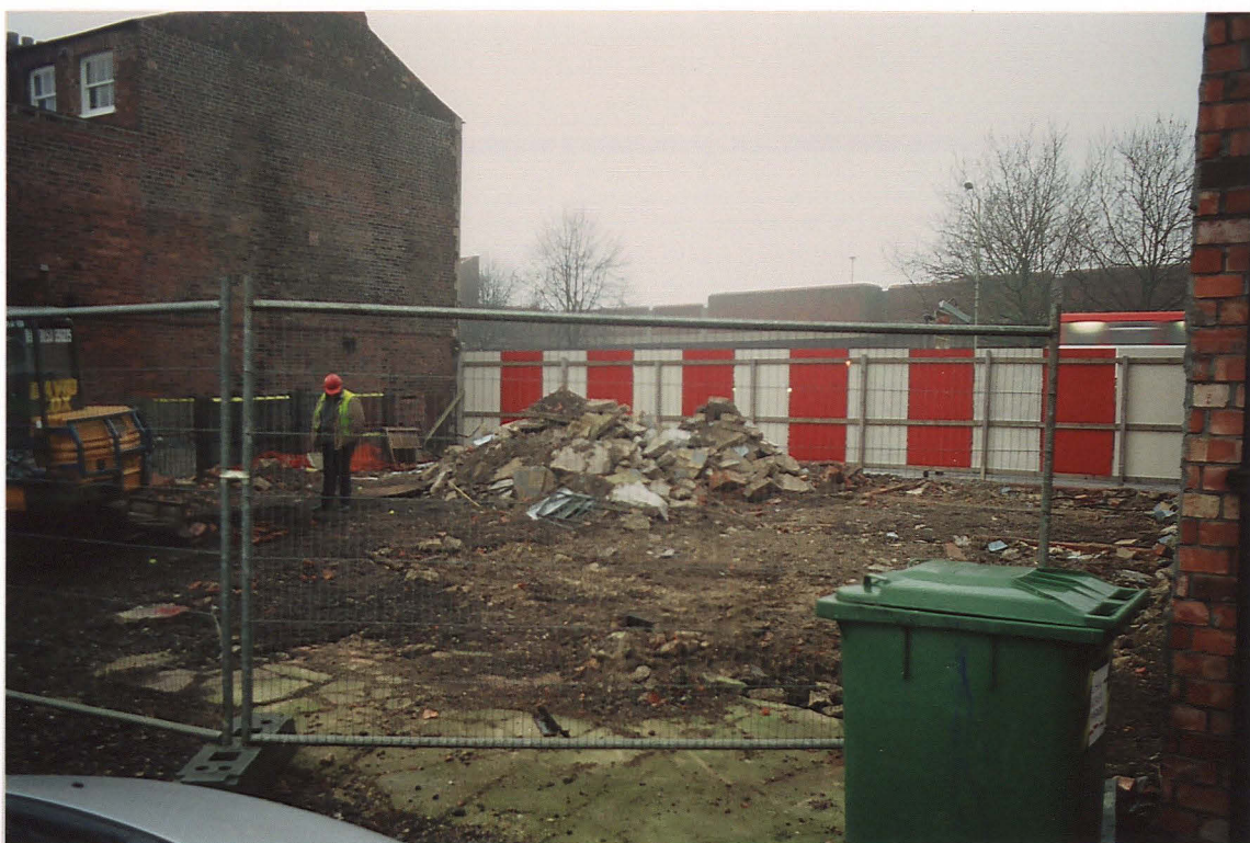
PI.13 General view of southern monitored area. Looking south west.
