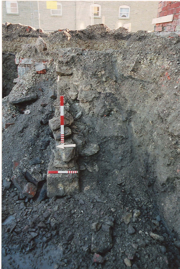
PI. 5 Wall 235. Looking east. Scales 0.50m. Vertical scales 0.50m, horizontal scale 0.30m.
