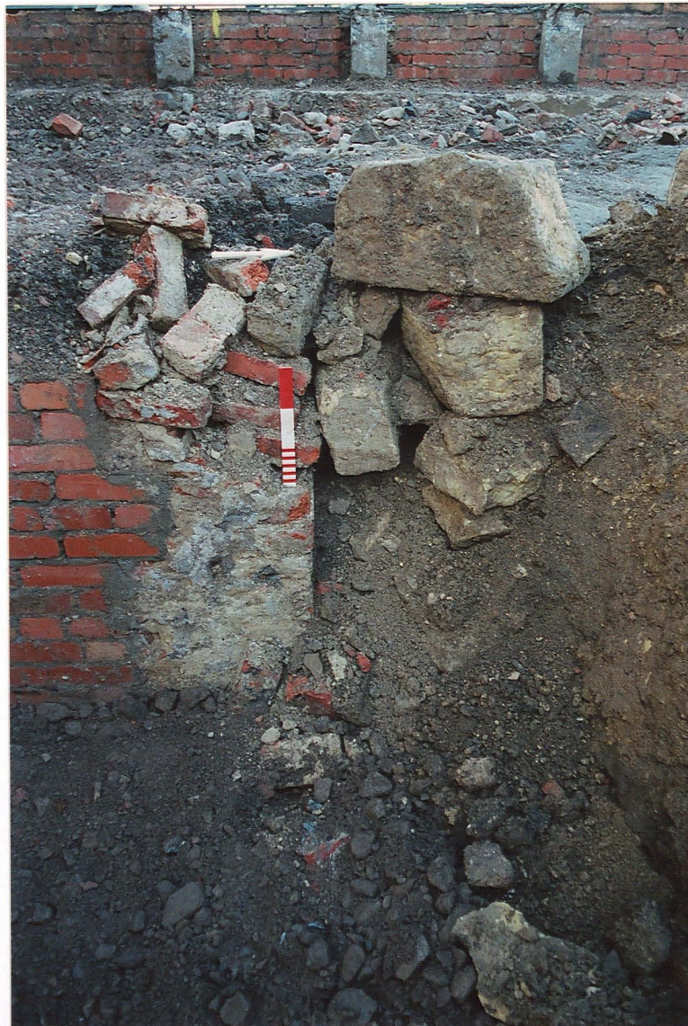
Pl. 3 Wall 234. Looking west. Scales 0.50m.
