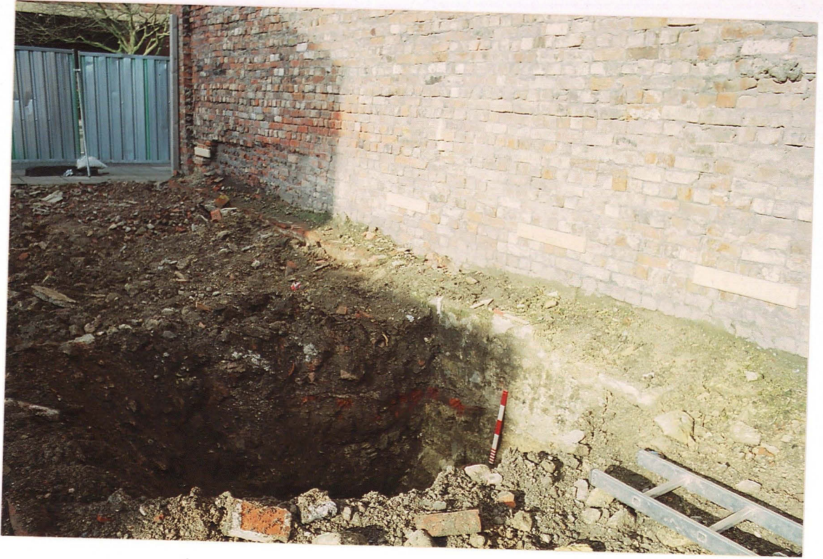
Pl.14 Western extent of wall 223. Looking west north west. Scale 0.50m.
