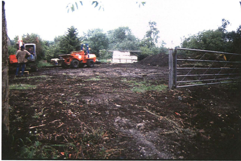
Plate 1 - General view of the site looking northwest
