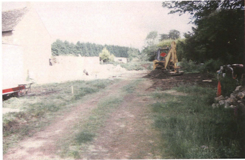
Plate 1 - General view of the site, looking north
